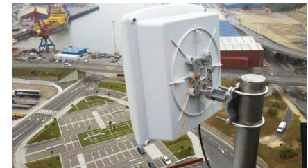
Wireless remote control system to manage the traffic lights at train crossings in Bilbao harbor.
